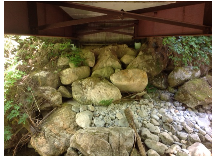
Right Bank Abutment when facing downstream
