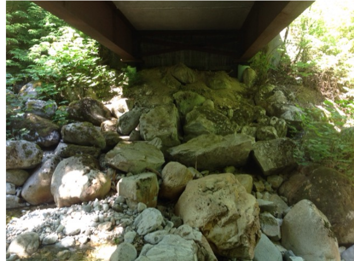
Left Bank Abutment when facing downstream
